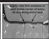
Continue around corner . At floor, leave protective backing to wall side. Work across floor with firm pressure up and down each rib. Then peel backing off wall side and apply pressure to it. Next continue with both seals up box. Stop at box contour near top. Leave adhesive protectors on- mark and cut seal to length for top and V-cut - as at top of other side -then finish adhering.
