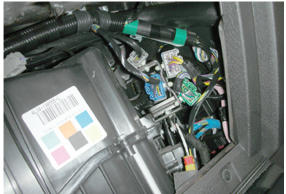
Wiring bundles after access panel is removed.
