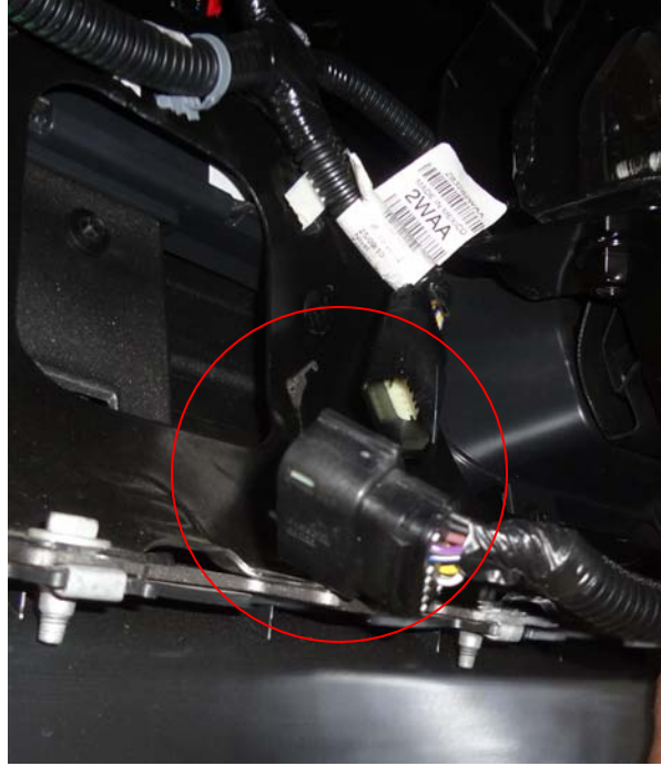
Figure 3(electrical harness disconnected)
