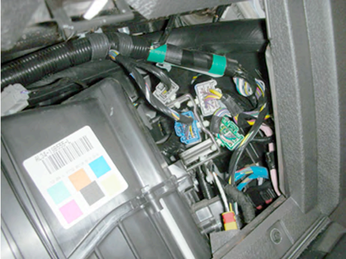
Wiring bundles after access panel is removed.
