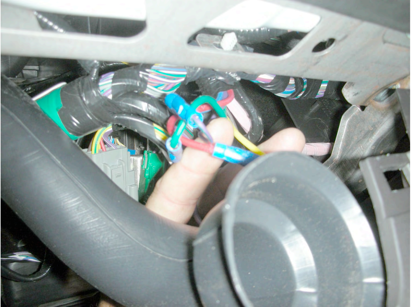
Mated wiring using butt connectors to show detail
