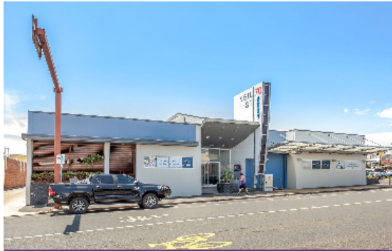
70 Neil Street, Toowoomba City
