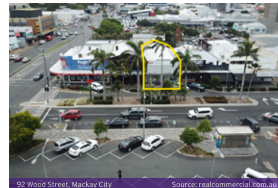
92 Wood Street, Mackay City
