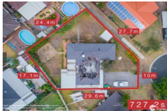
A fire damaged house in Woodbine (Source: CoreLogic)
