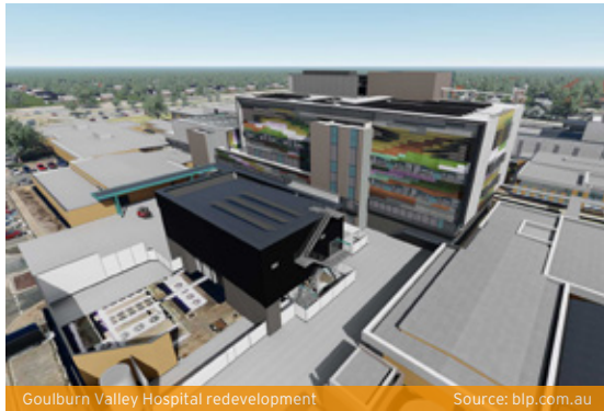
Goulburn Valley Hospital redevelopment Source: blp.com.au
