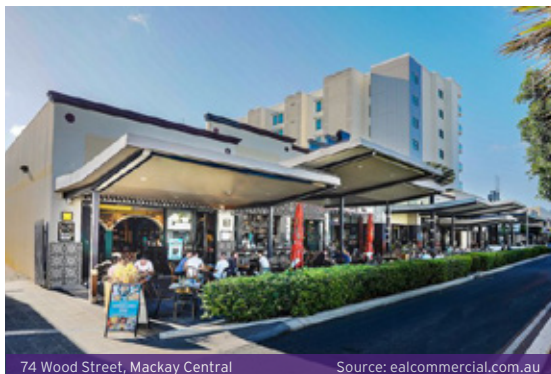
74 Wood Street, Mackay Central
