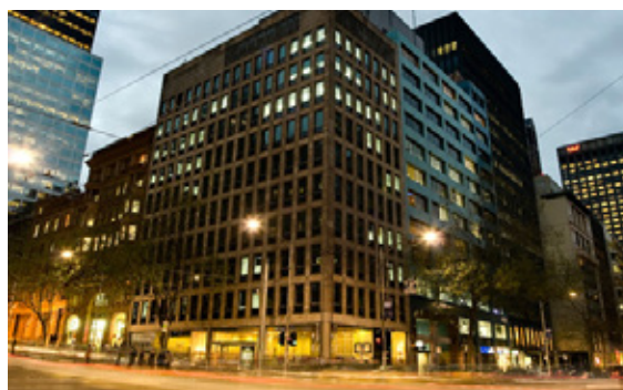
454 Collins Street Image (source: Metaxas Architects)
