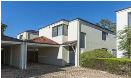
Figure 9 : Beveridge Street, Bentley Source: CoreLogic
