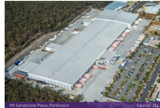
99 Sandstone Place, Parkinson
