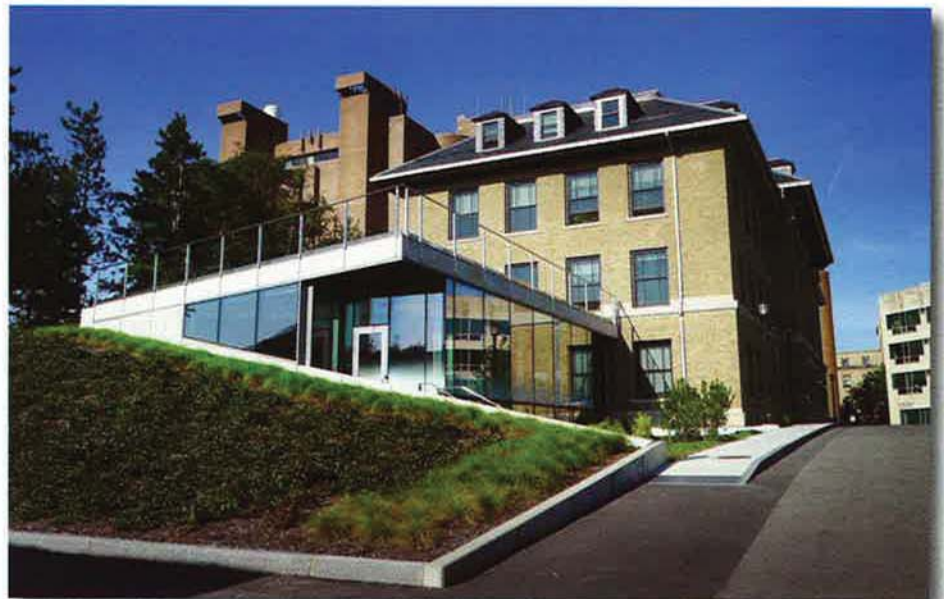
A 1,700-square-foot addition to Fernow Hall at Cornell University in Ithaca, N.Y., incorporated a green roof and rain garden onto the property.
