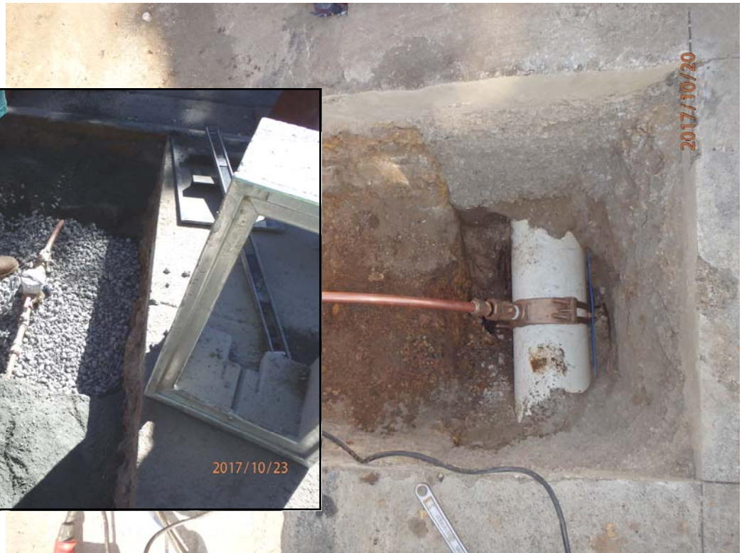
Oct 19 thru Oct 30, 2017—Meter connections (South Road)
