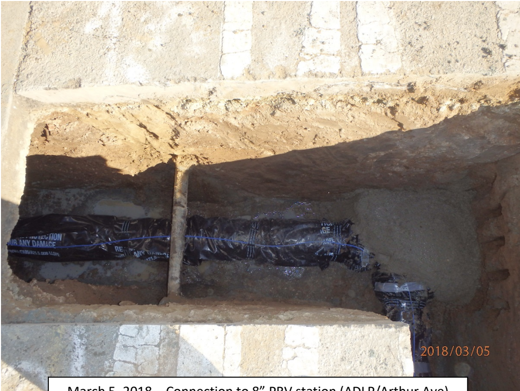
March 5, 2018 – Connection to 8" PRV station (ADLP/Arthur Ave)
