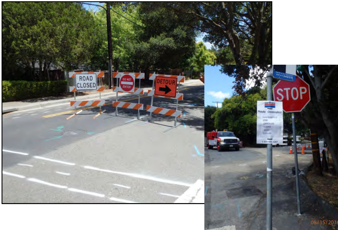
July 15, 2016 - Road closure (traffics were detoured round the construction zoon)
