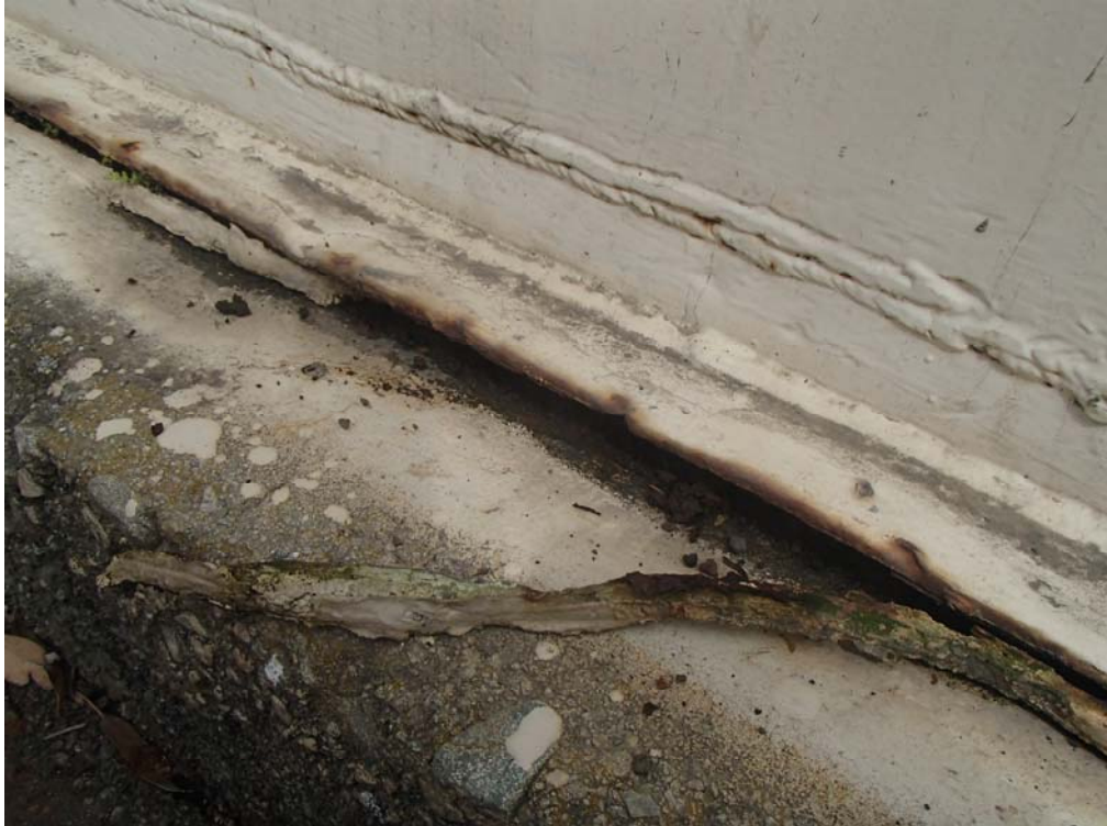
Photo 9: Corroding Tank Bottom Plate
