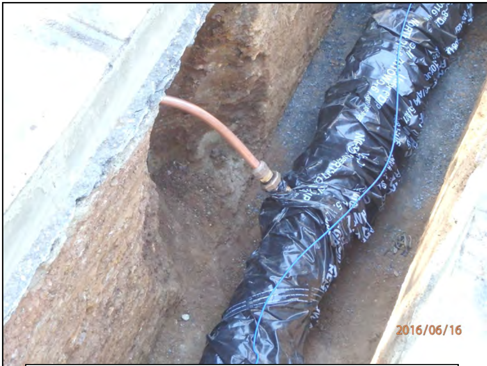
June 16, 2016 - Installation of water service lines
