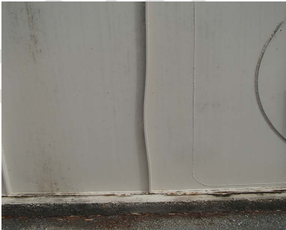
Photo 4: Misaligned Tank Stiffener Plate
