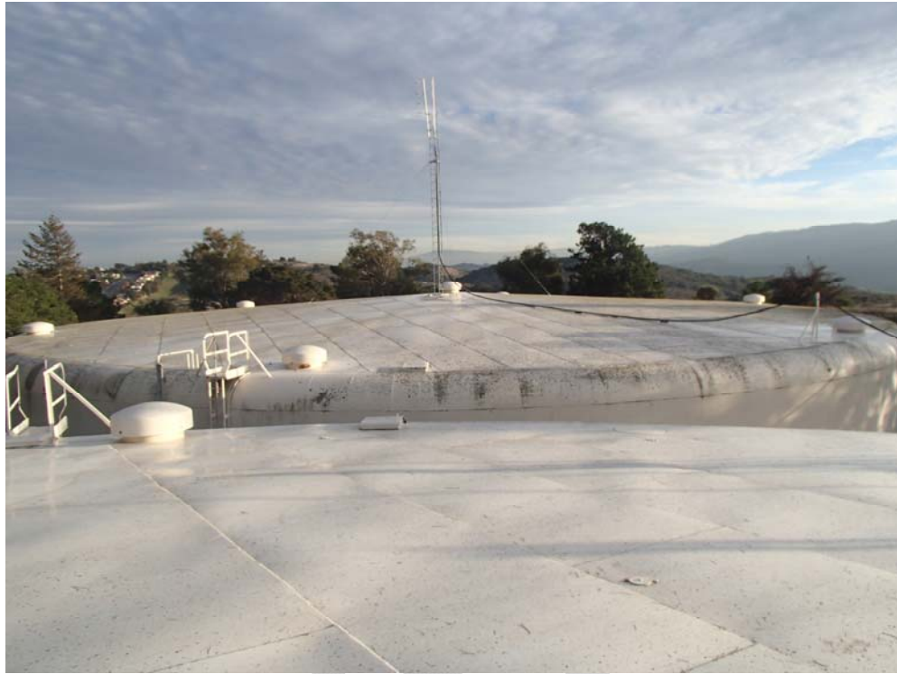
Photo 5: Roof of Hallmark Tanks
