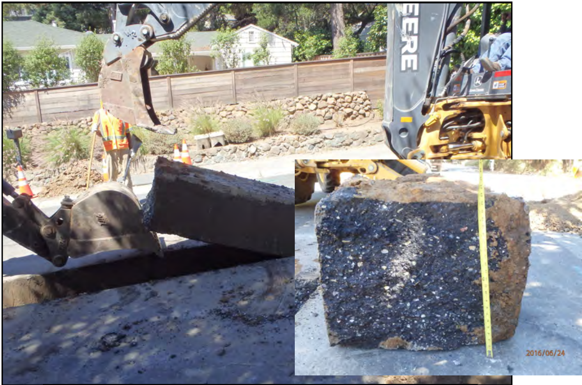
June 26, 2016 - 21" asphalt thickness at Mezes Ave
