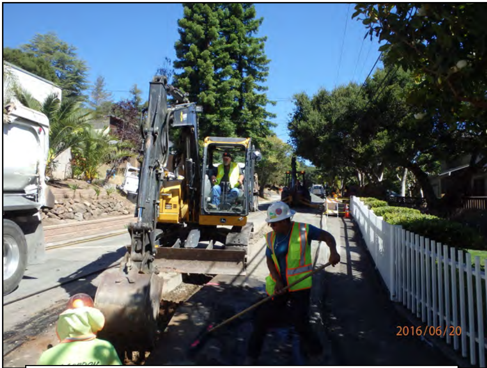
June 20, 2016 - Water main installation (trenching)
