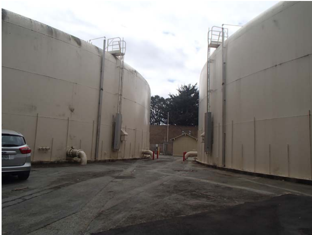
Photo 1: Exterior of Hallmark Tanks
