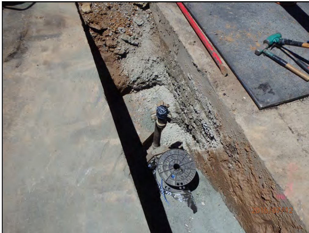
July 12, 2016 - Temporary blow-off at end of the water main prior to tie-ins
