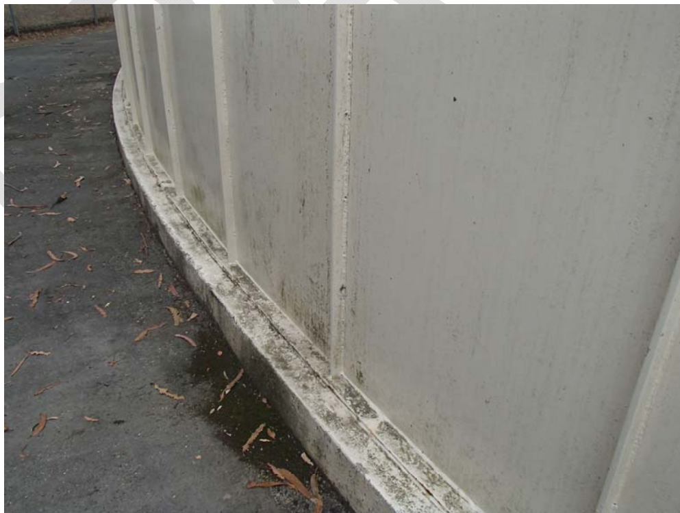
Photo 2: Reinforced Concrete Ringwall Foundation
