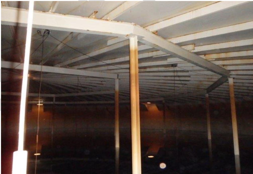
Photo 8: Interior Roof Framing of Hallmark Tanks
