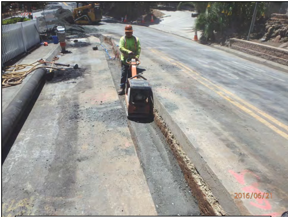
June 21, 2016 - Compaction
