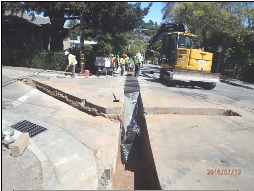
July 19, 2016 - 4 valve set at Lyon Ave
