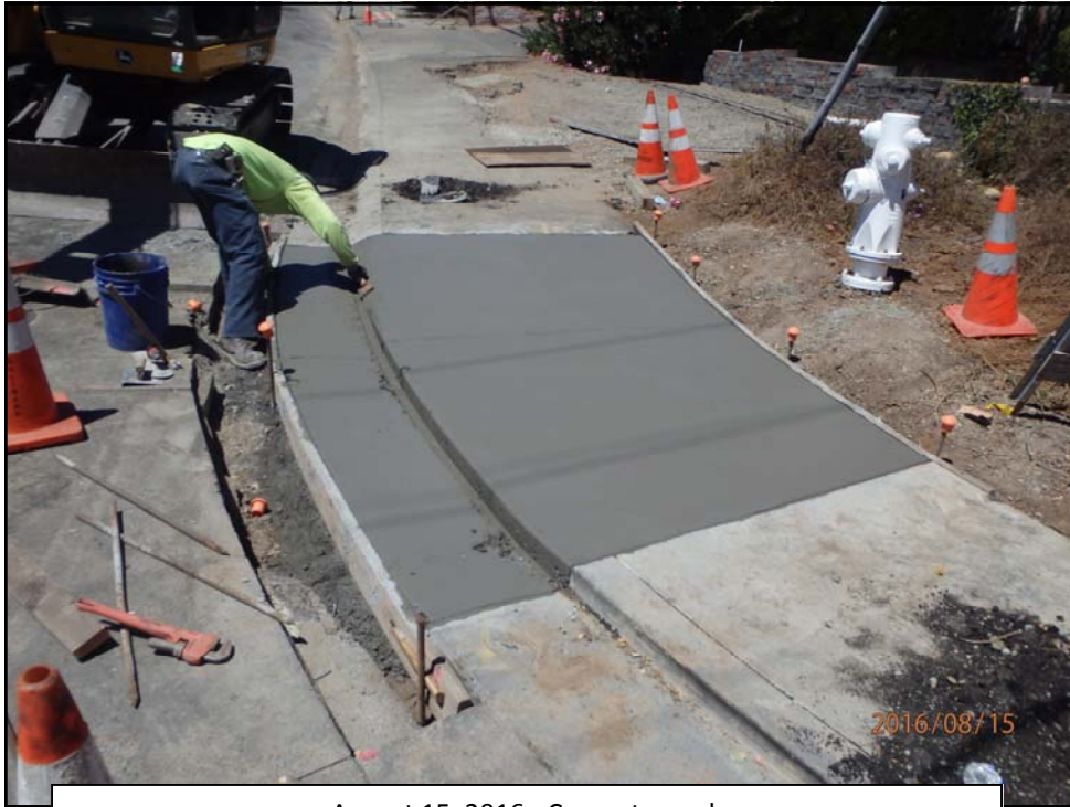
August 15, 2016 - Concrete work
