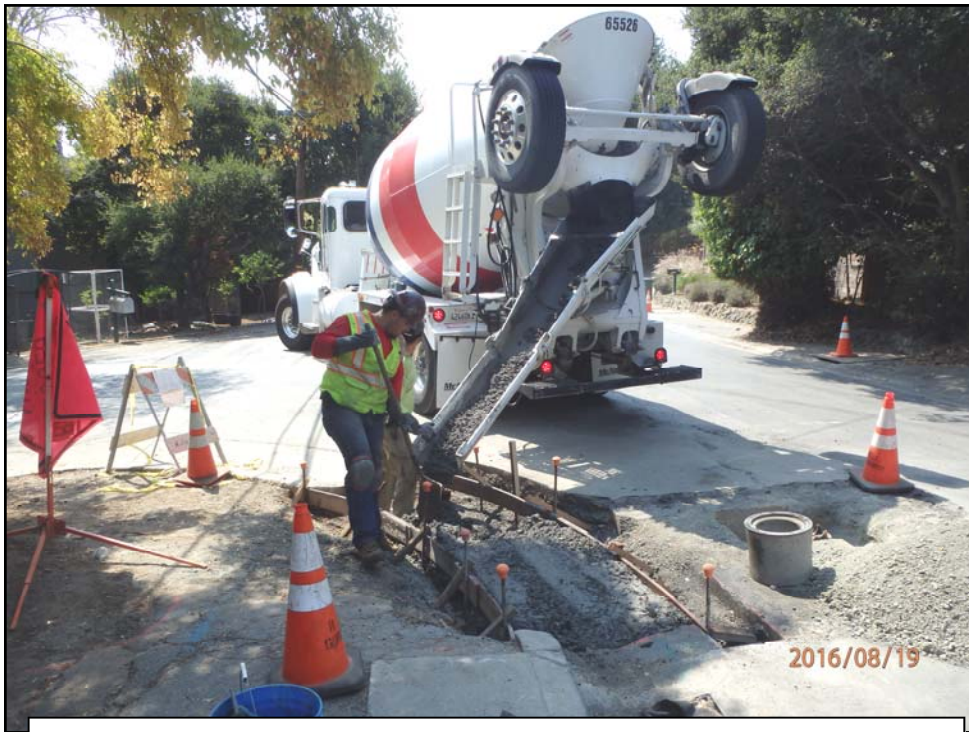
August 19, 2016 - Concrete work
