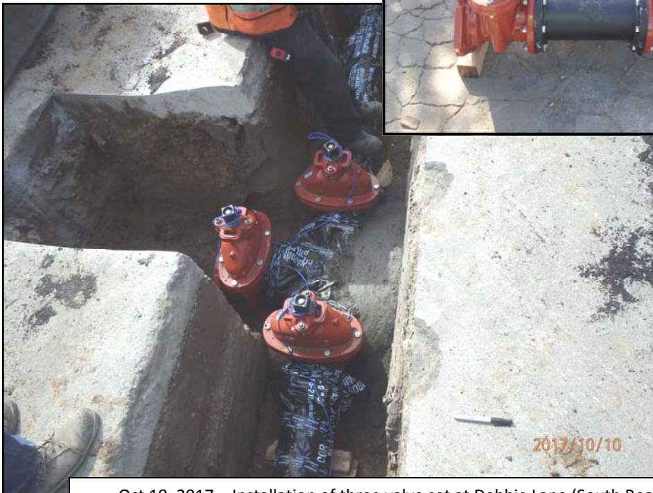
Oct 10, 2017 - Installation of three valve set at Debbie Lane (South Road)
