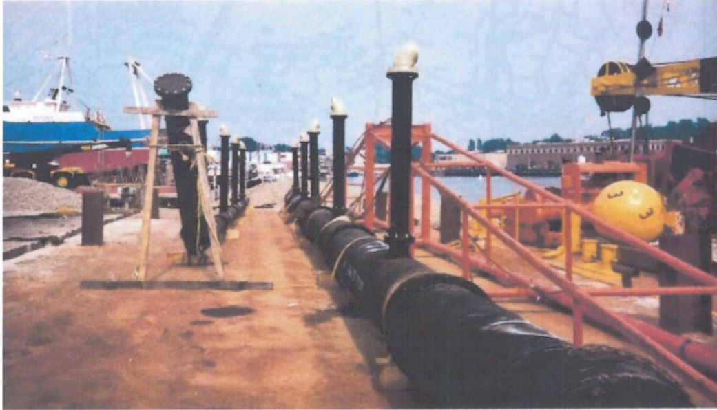
Fig 2. Outfall diffuser prior to installation.
