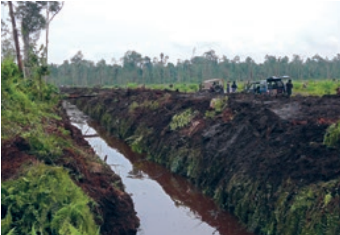
26 July 2007, Riau, Indonesia: Recently cleared peatland and drainage canal on very deep peat in a Duta Palma concession. ©Greenpeace
