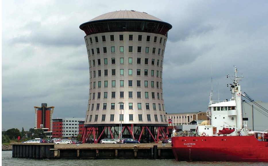
FIG. 26 Mammoet would later transport a complete office building over water from Zwijndrecht to Dordrecht, 30 km
