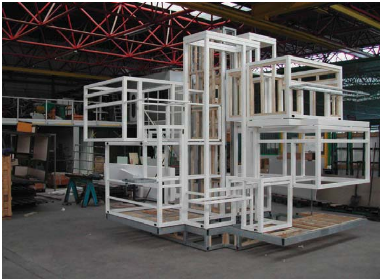
FIG. 63 Total assembly of the steel skeleton.
