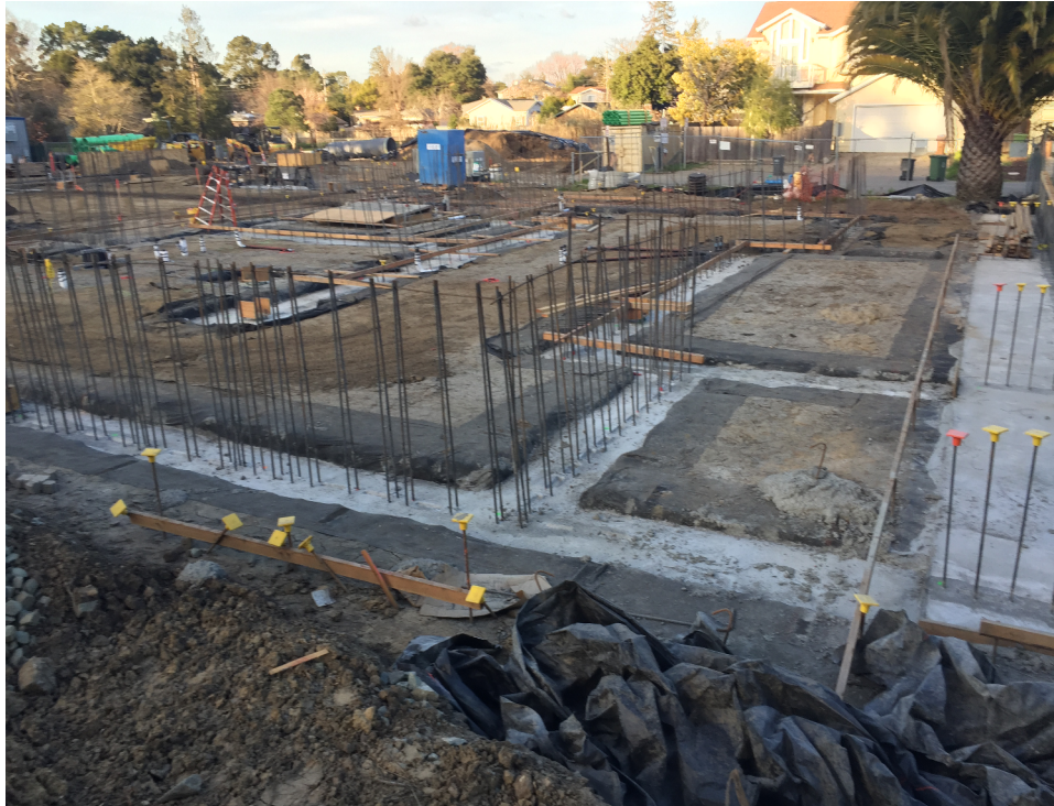
January progress pictures for Fire Station 57
