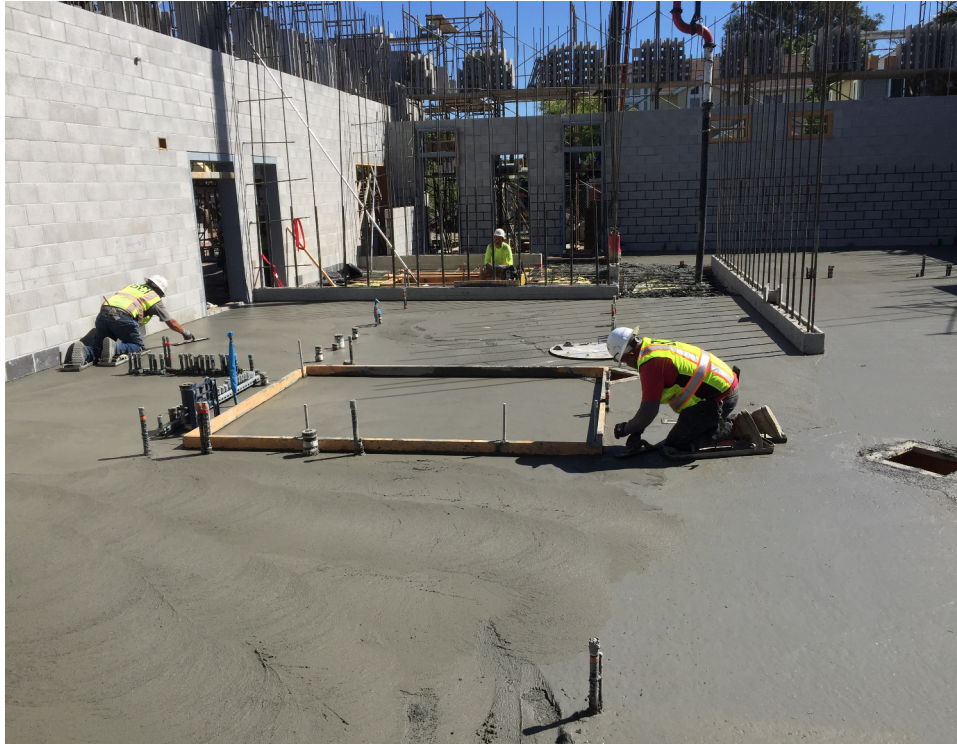
May progress pictures for Fire Station 57
