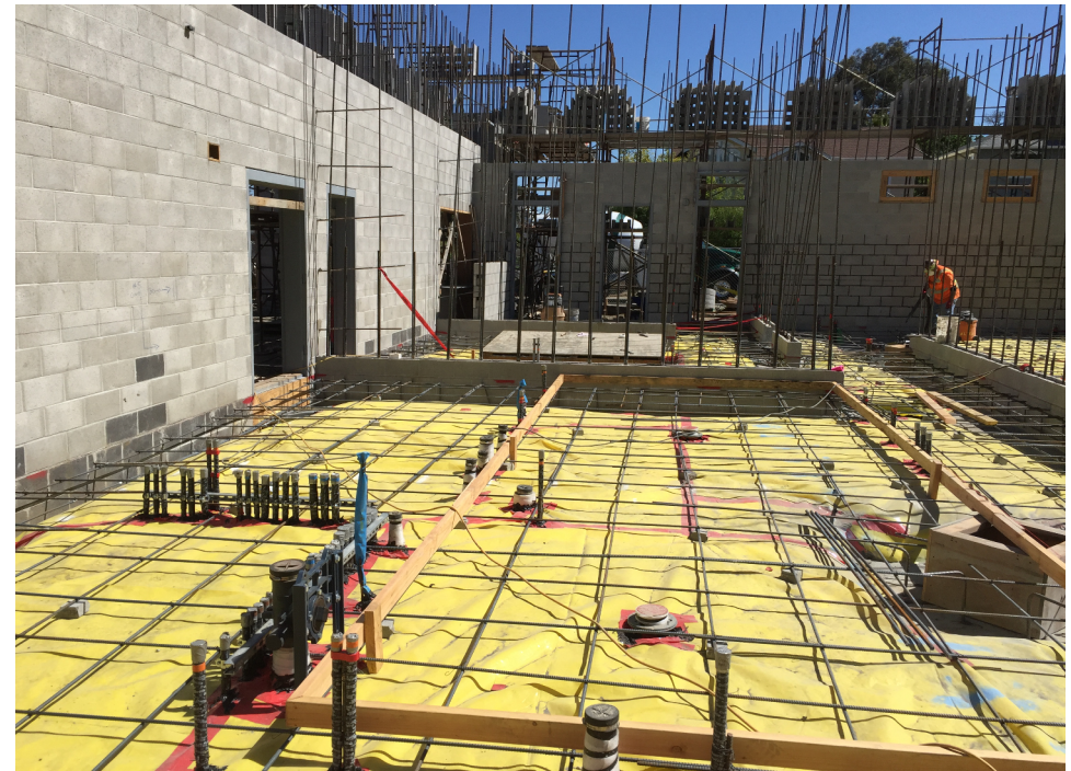
May progress pictures for Fire Station 57
