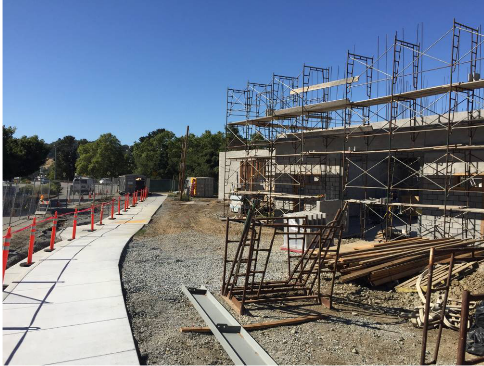
June progress pictures for Fire Station 57
