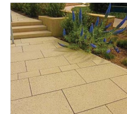
CONCRETE UNIT PAVER 24" X 48"
