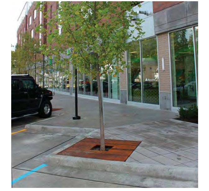
CONCRETE SIDEWALK WITH TREE GRATE
