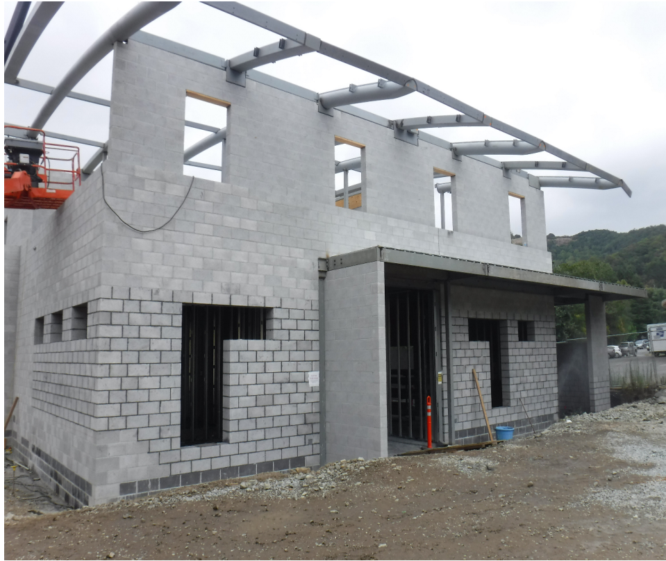
August progress pictures for Fire Station 57
