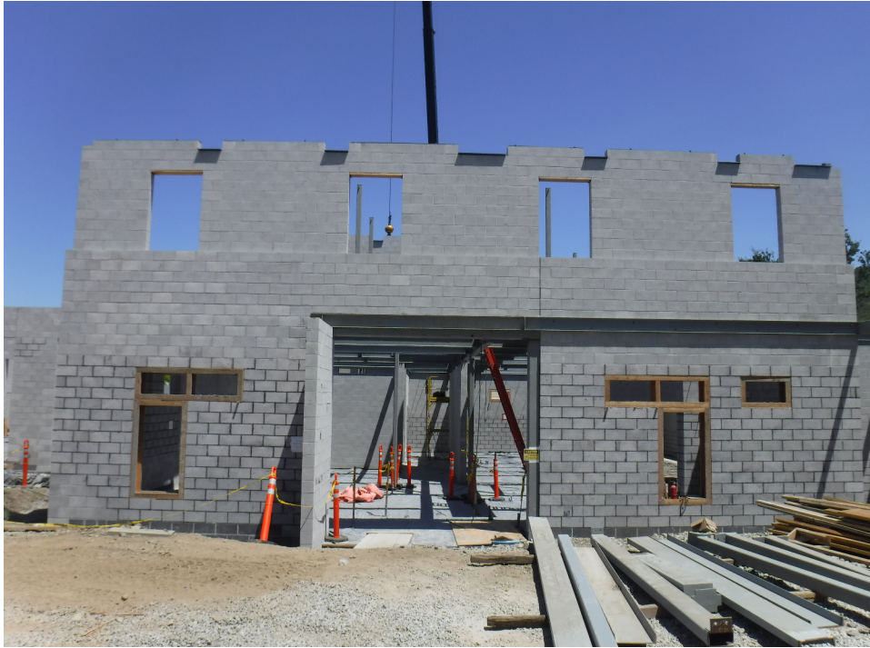
July progress pictures for Fire Station 57
