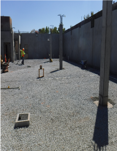
August progress pictures – Under Slab rock and water proofing at the basement and App. Bay
