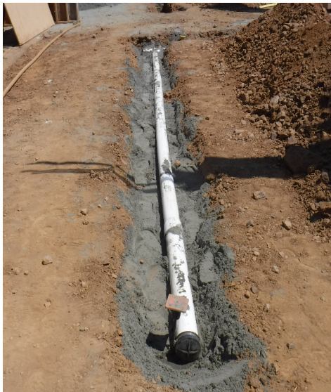
August progress picture – Under Slab Utilities (Storm Drain and Sewer)
