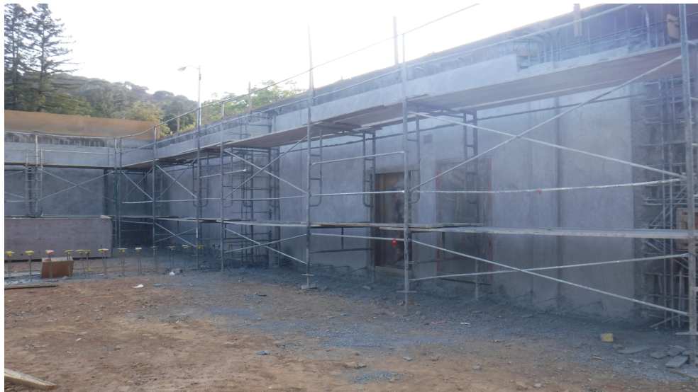
July progress picture – Shotcrete Wall and Scaffolding along C-Street
