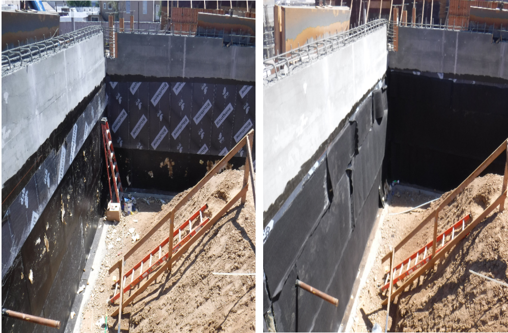
July progress pictures – Water Proofing of the Basement along 5 th Avenue
