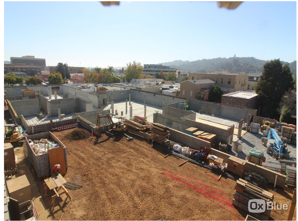
September progress picture – Overview of project site progress.
