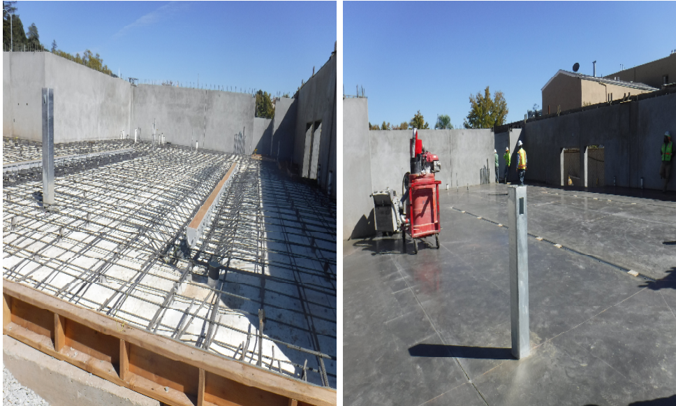
September progress picture – The App. Bay room before and after the concrete pour
