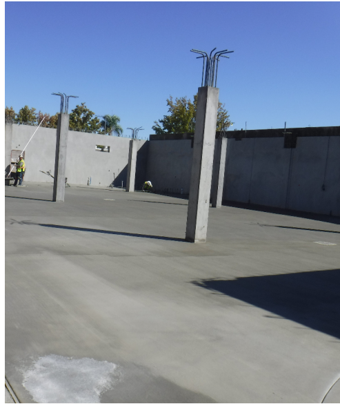
September progress pictures—placement of rock, water proofing and concrete at the basement level parking
