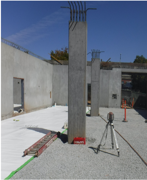
September progress pictures—placement of rock, water proofing and concrete at the basement level parking
