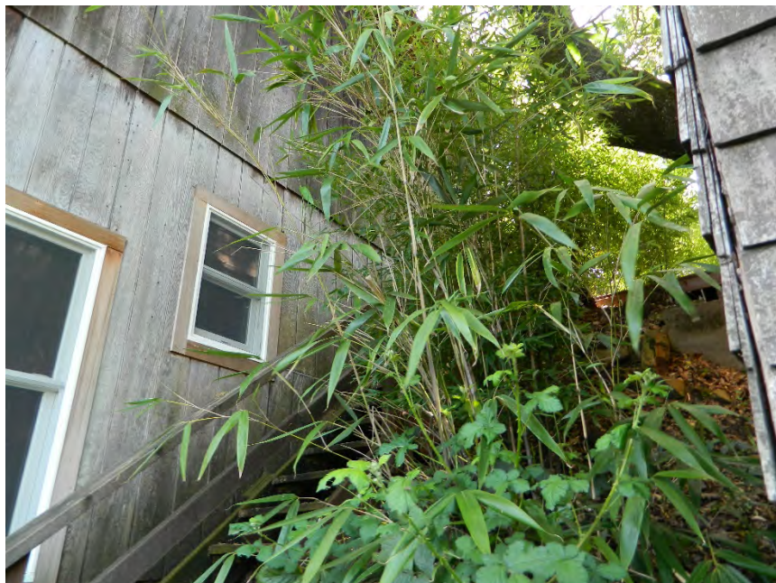
Photo showing the north elevation, facing west/southwest.
