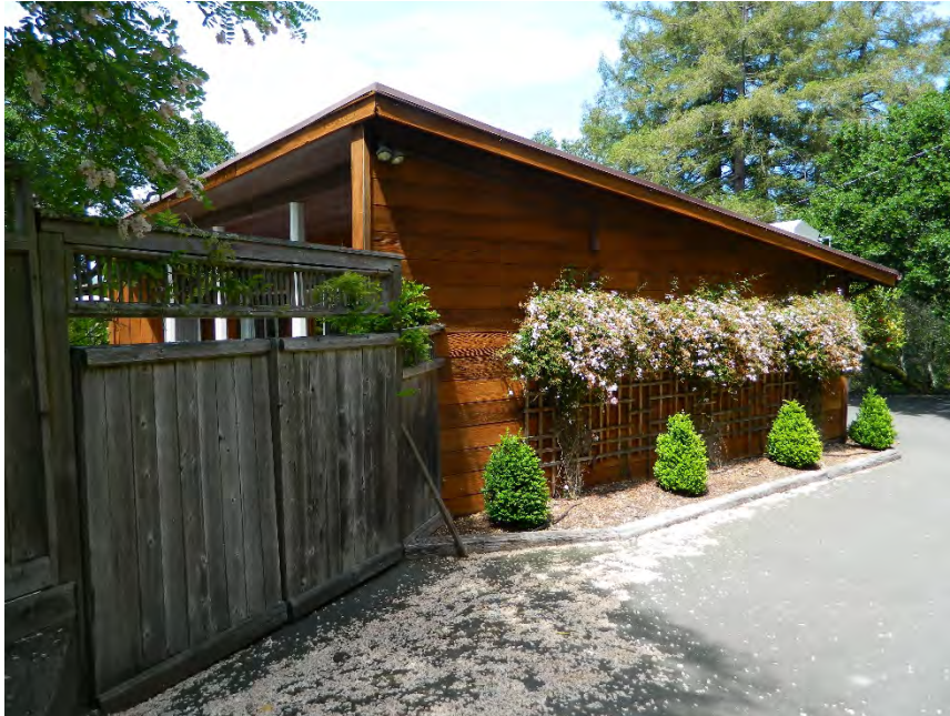
Photo showing the southeast elevation, facing north.
