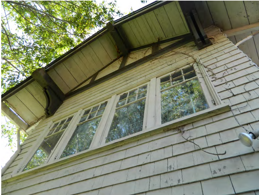
Photo showing the north elevation "ground floor" gable with knee braces and gable timber detail.
