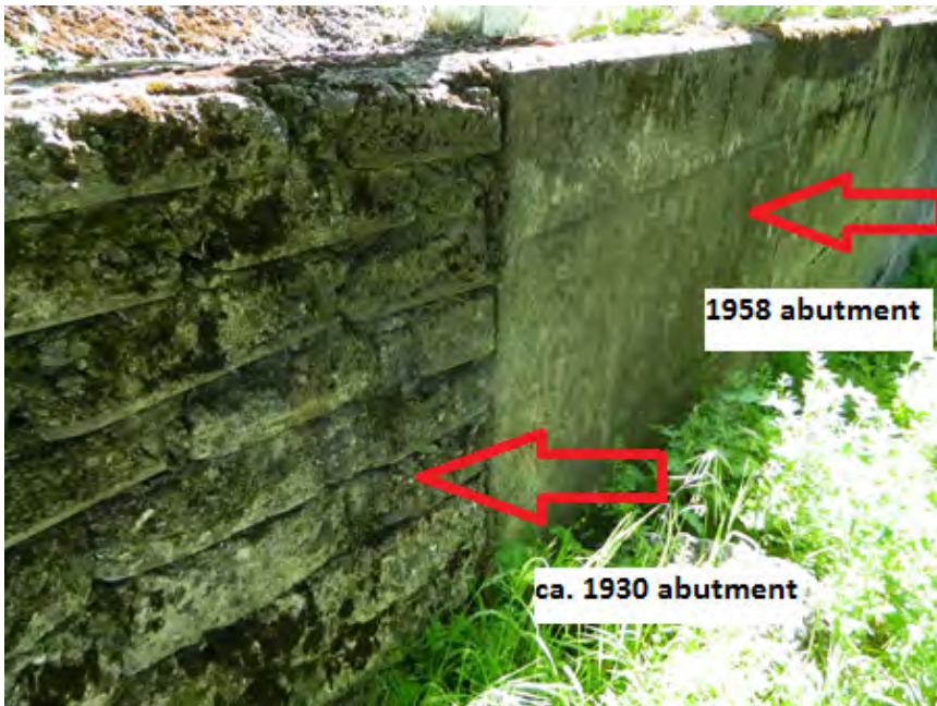
Photo showing ca. 1930 abutment and the 1958 abutment.
