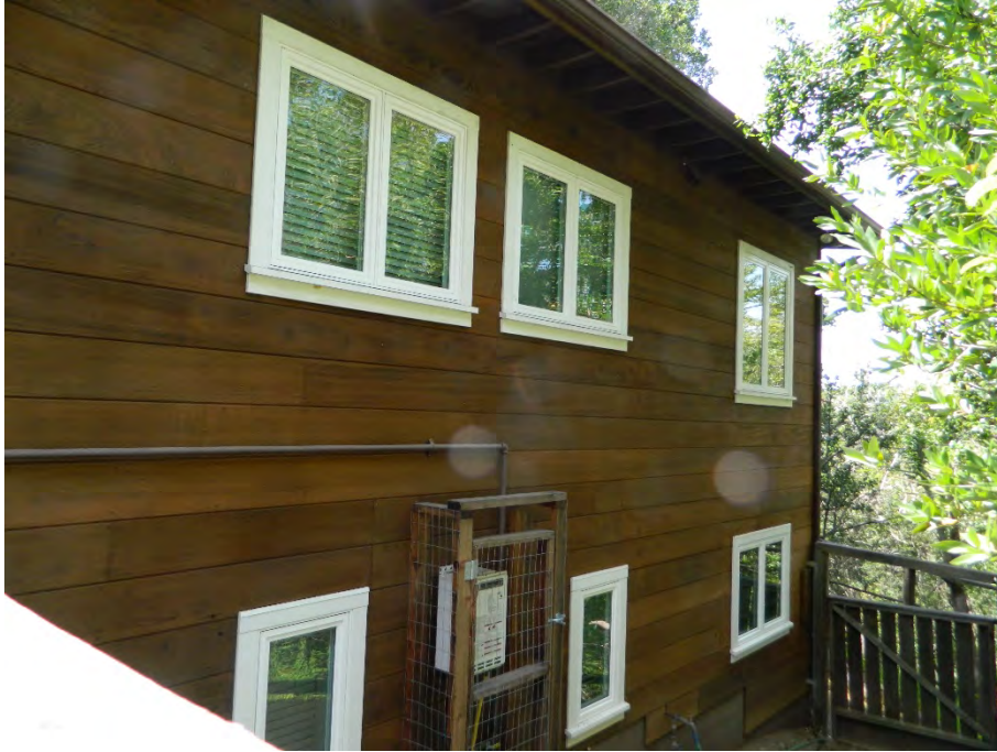
Photo showing the northeast elevation, facing west.
