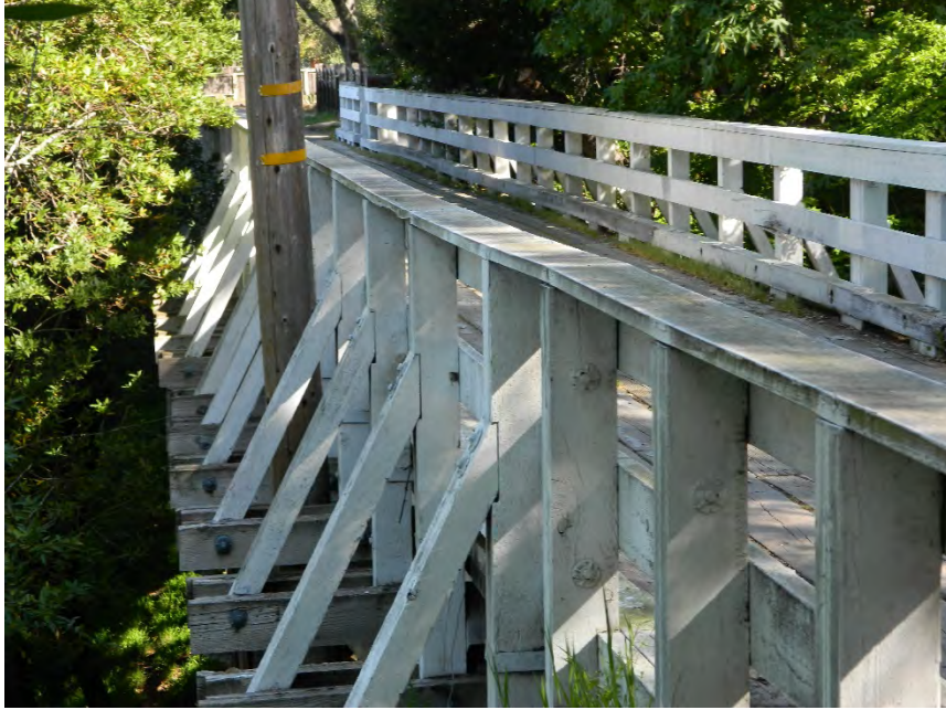
Photo showing the east side at the north approach to the bridge, facing south.
