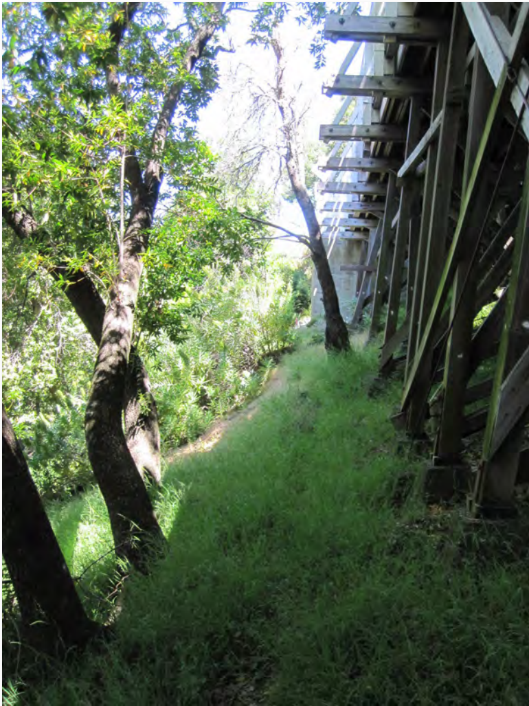
Photo from below bridge, facing north.
