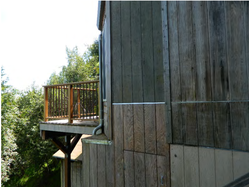
Photo showing the north elevation, facing east/southeast.
