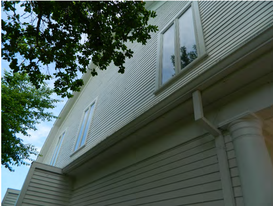
Photo showing the north elevation, second story overhang.
