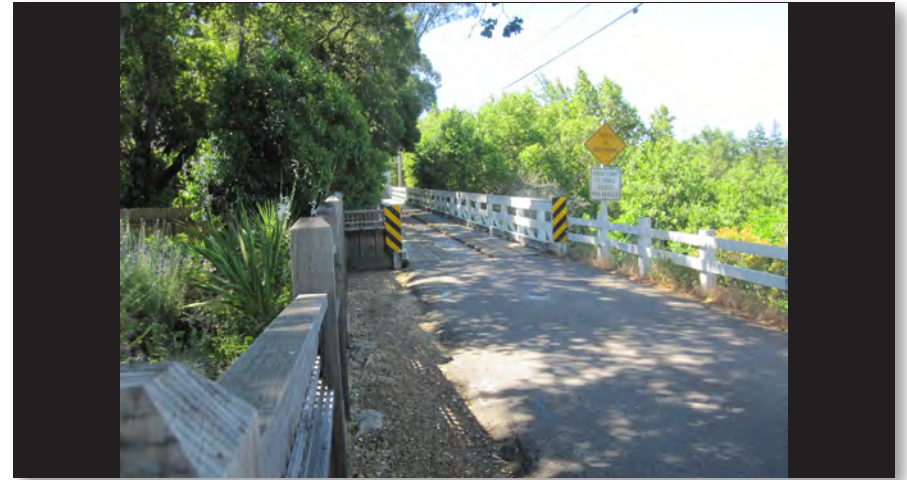
Photo of north end of bridge, facing south.
