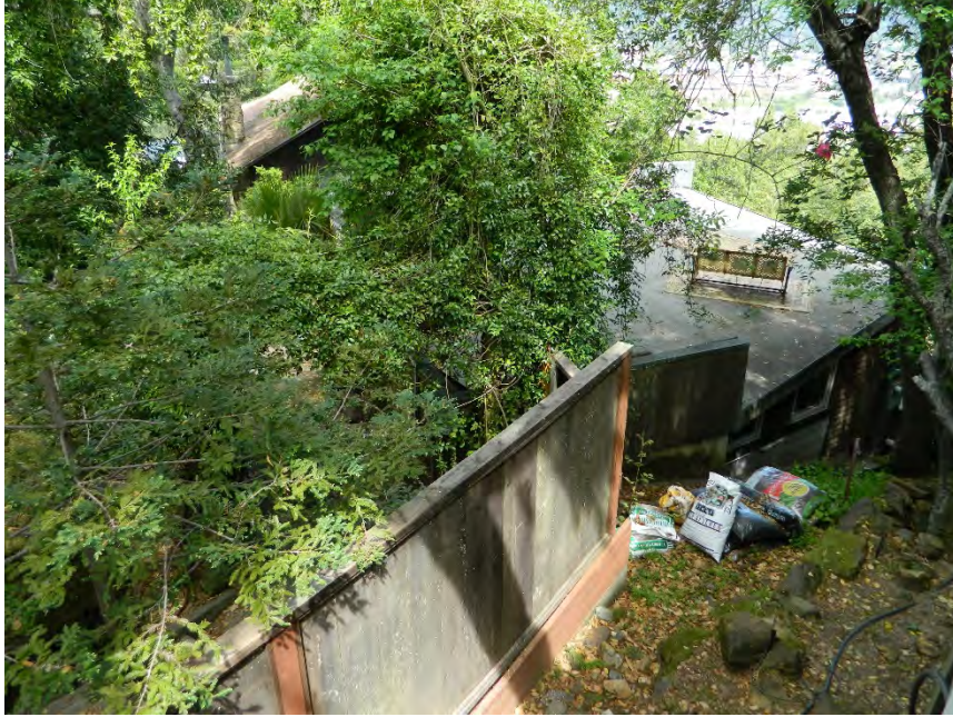
Photo showing the south elevation, facing north/northeast.
