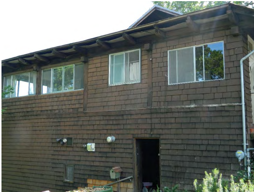
Photo showing the north elevation, facing east/southeast.
