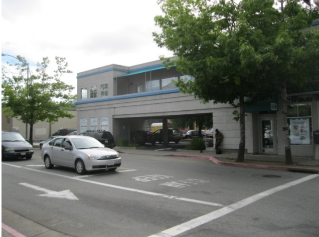
2. East Facade of Building
