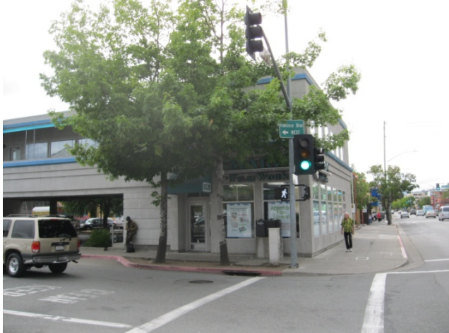
1. North and East Facades of Building
