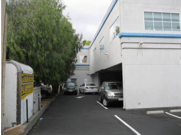
5. West and South Facades of Building
