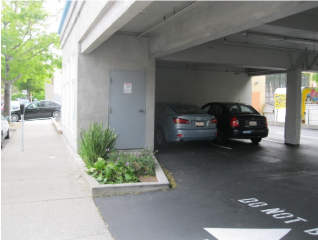
7. Ground Floor Parking Area, East Entrance
