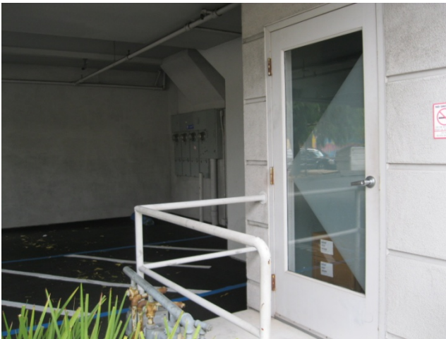
9. Ground Floor Parking Area, Stairwell Entrance
