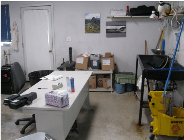
15. 2nd Floor Photo Chemical Storage and Sink, Minor Staining Visible on Floor
