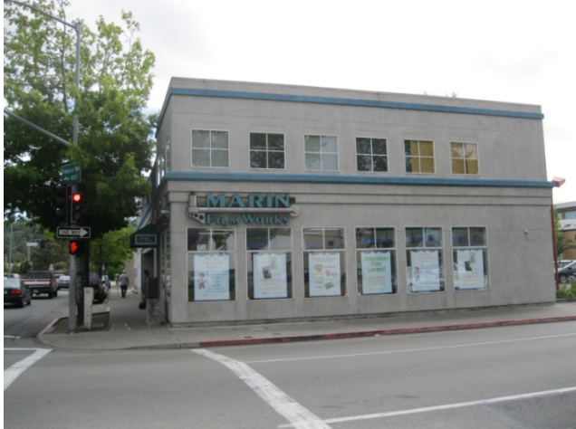
3. North Facade of Building
