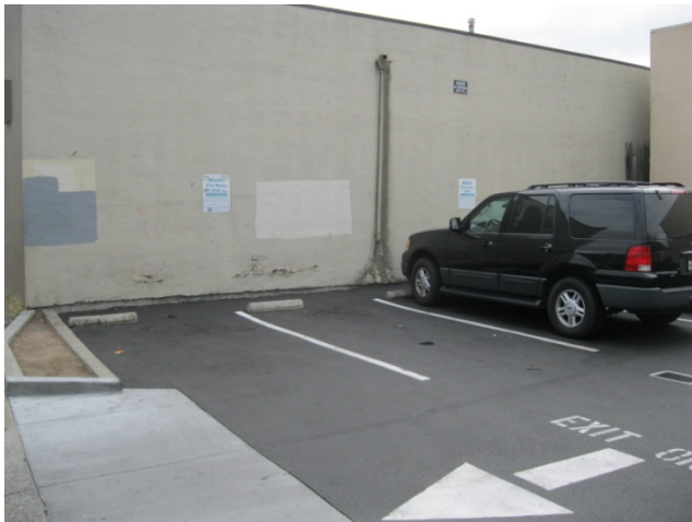
21. Adjoining Building to South of Subject Property Parking Area
