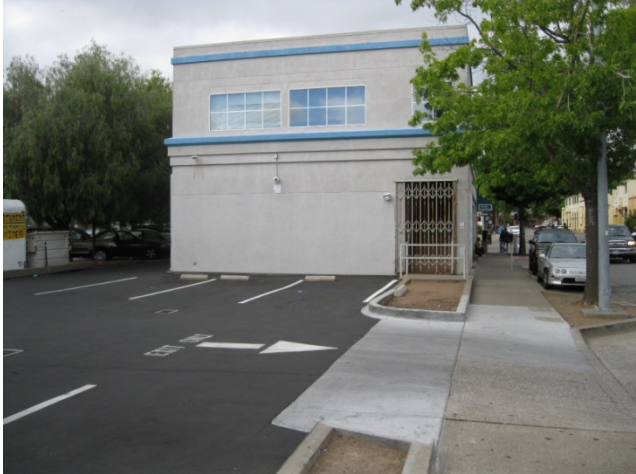
6. South Facade of Building
