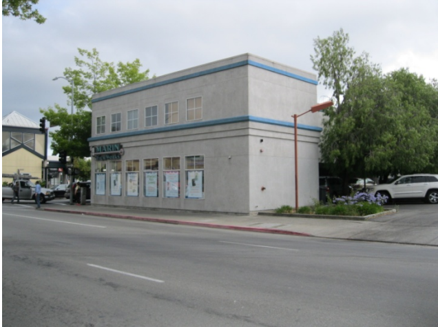
4. North and West Facades of Building
