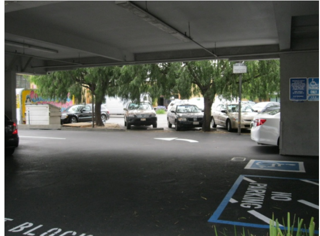
8. Ground Floor Parking Area, West Entrance
