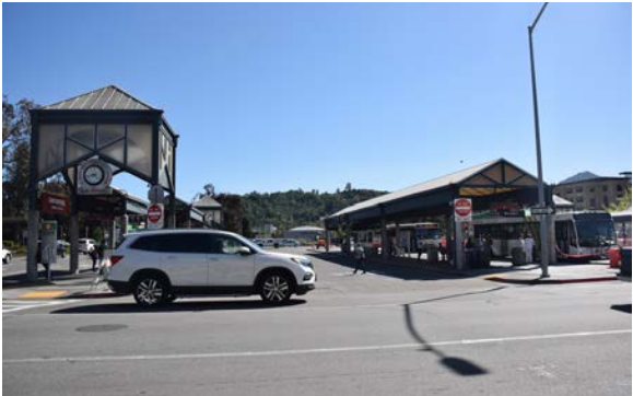
Downtown San Rafael Transit Center, a regional hub
