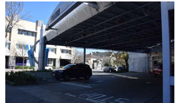
An example of poor frontage: the facade is set back and has no active relationship with the adjacent street.
