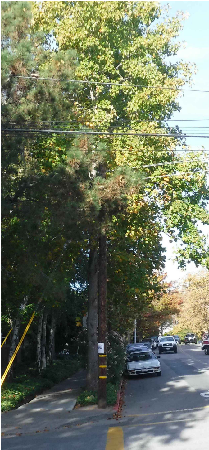
EXISTING POLE PHOTO
