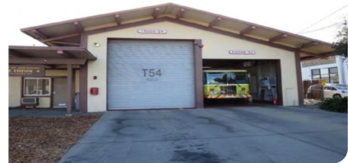
Front of Fire Station 54
