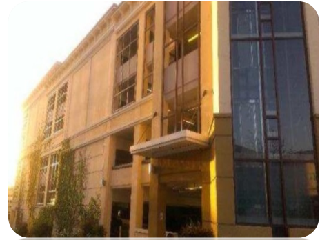
Third and C Parking Structure
