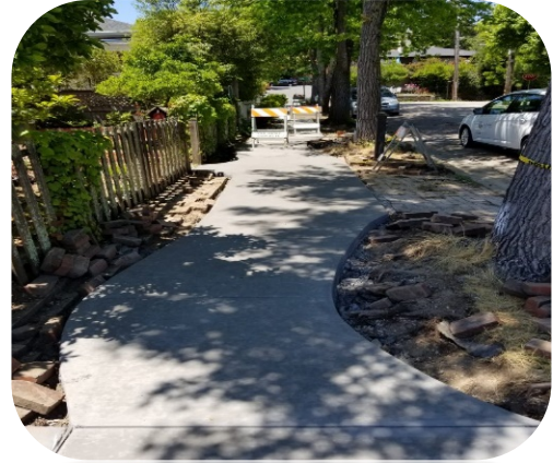
Bayview St. repaired by constructing the sidewalk around the tree
