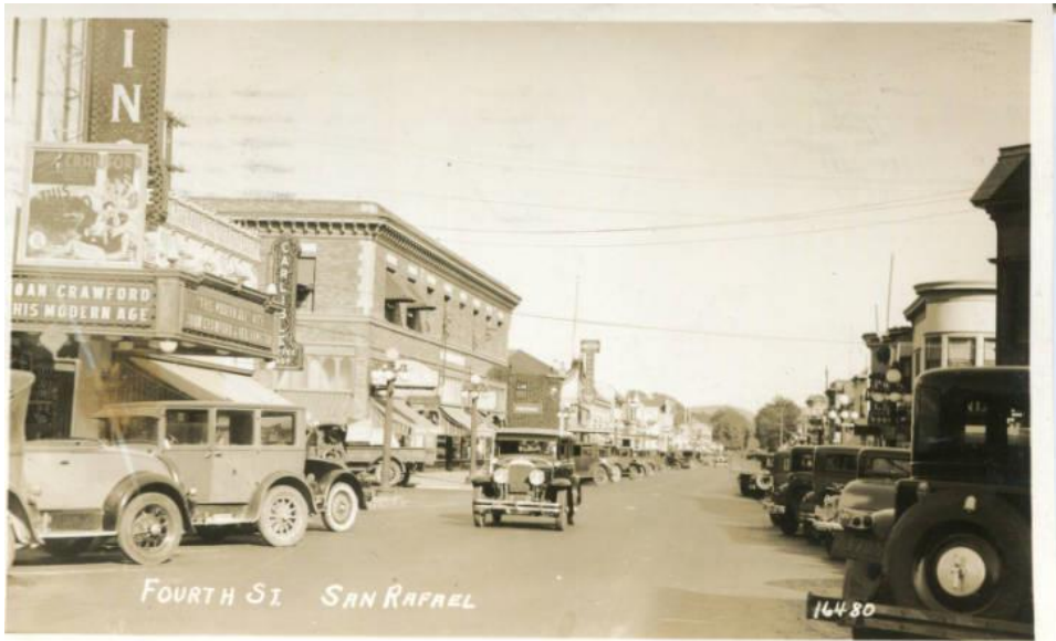
Figure 7: View of Fourth Street looking east, 1932. Anne T. Kent California Room.
