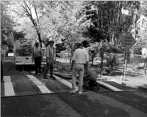
A Public Works crew installs a speed hump to slow neighborhood traffic.
