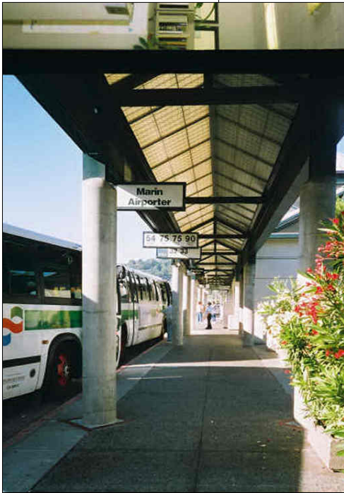
The Bettini Transportation Center is a multimodal transit hub with services connecting San Rafael to San Francisco, the East Bay, and the North Bay.
