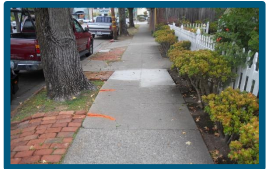
Displaced sidewalks in San Rafael
