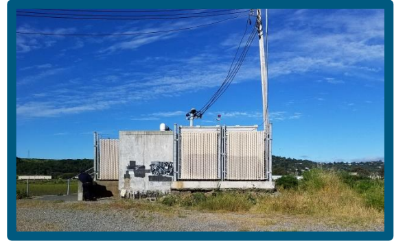
San Quentin pump station
