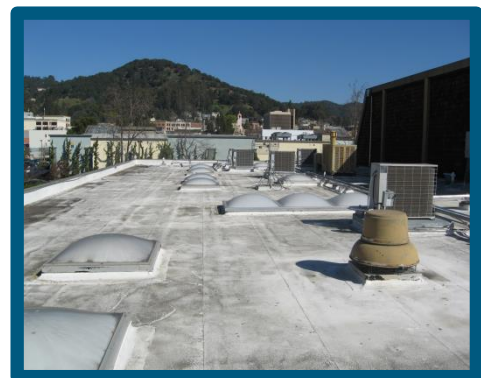
B Street Community Center Roof
