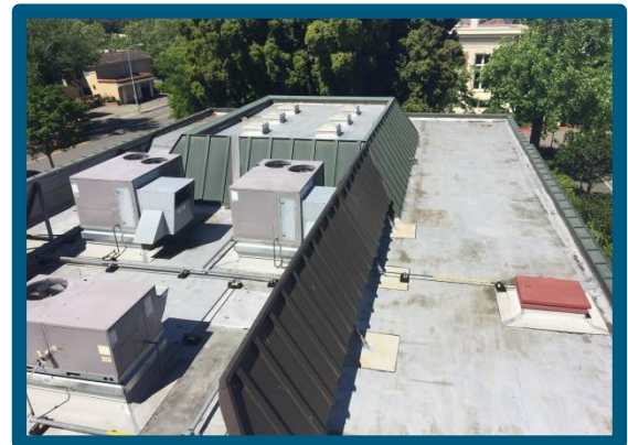
City Hall roof from above
