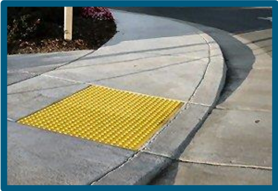
An ADA-accessible sidewalk curb ramp
