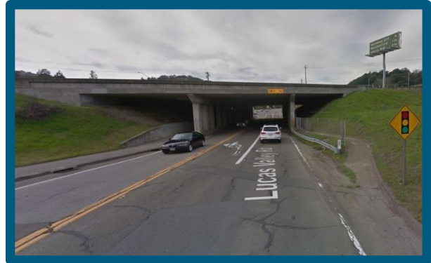
Smith Ranch Road under Highway 101
