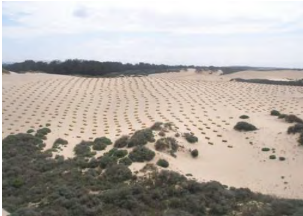
Figure 6-10. Top: A part of the 15-acre wind fencing array installed at Oceano Dunes SVRA in 2014. Note monitoring equipment at trailing edge of array. Bottom: The 30-acre straw bale array installed outside the Oceano Dunes SVRA open riding and camping area in 2014.
