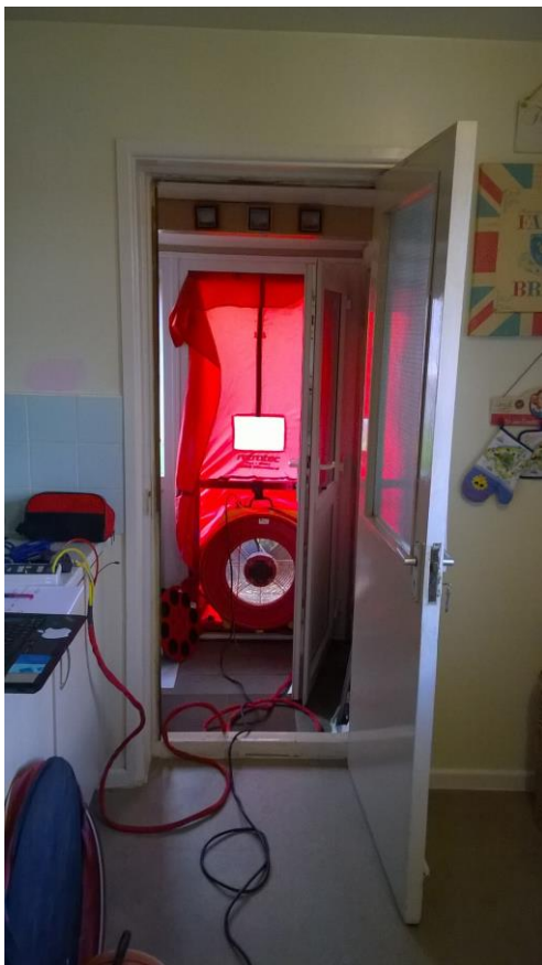
Door fan installation at House A
