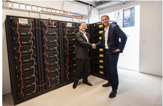
Figure 15: Evermore Battery System
