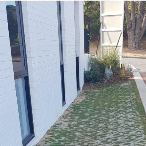
Figure 13: Section of Permeable Paving
