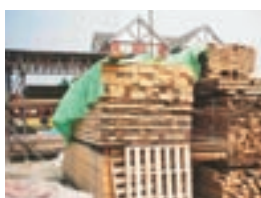
Reclaimed timber studwork delivered to site
