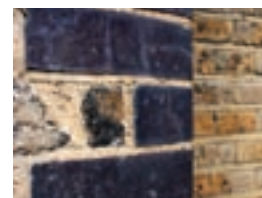
Staffordshire Blues and London Yellow Stock bricks due for reclamation on a London regeneration project
