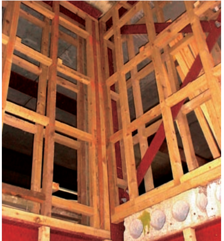
Timber studwork during construction
