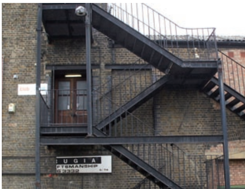
Re-use of staircase being investigated
