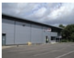
Building prior to demolition
