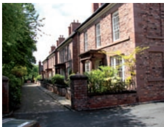
Reclaimed bricks used in redevelopment
