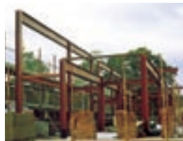
Reclaimed steel was used for the structure
