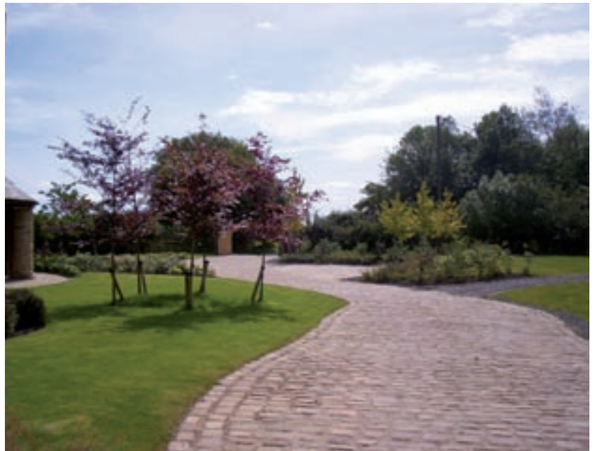
Completed areas of gritstone paving
