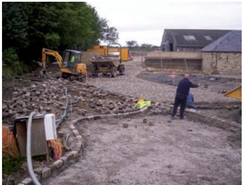
Laying of reclaimed gritstone setts
