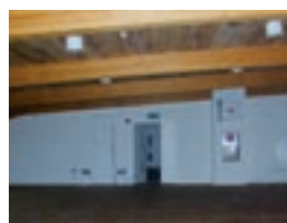
Function hall after completion
