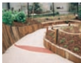
Ekki sleepers retaining wall up to the exit
