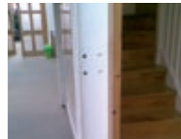
Staircase and partition wall
