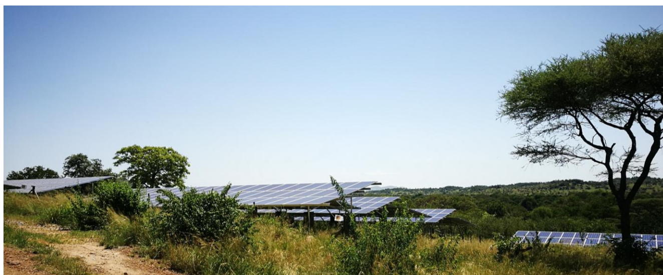
Image 5: 189kWp of photovoltaic panels nestled into the landscape at Faru Faru
