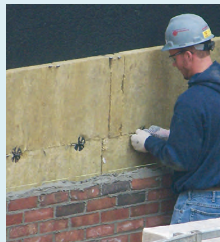
Easy-to-cut RainBarrier installs with common wall ties and insulation hangers.
