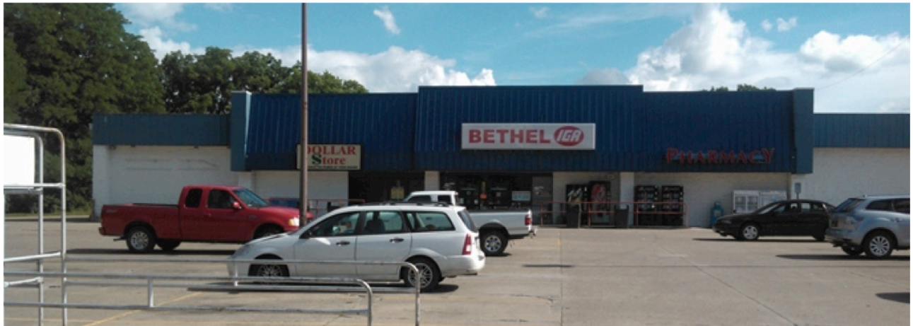
The outside of our location at 545 W. Plane St. Bethel, Ohio, before renovation (photo: Nadine Albenze-Smith, 6/1/15)
