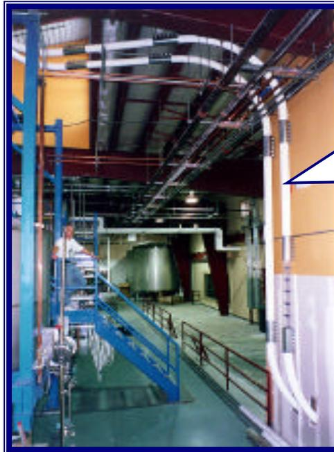
Super IV adapts to existing plant, by climbing a vertical interior wall.
