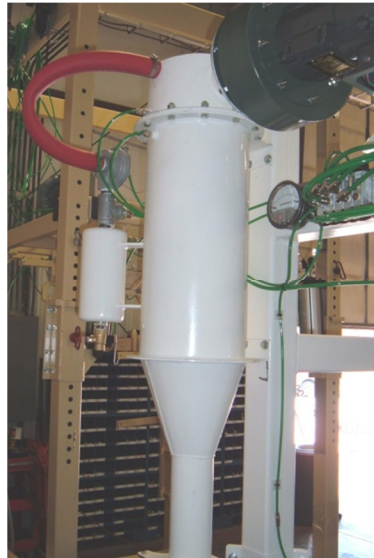
Self-contained dust collection systems return product back to process stream
