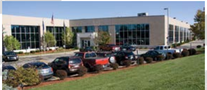
SWECO World Headquarters Florence, Kentucky, USA
