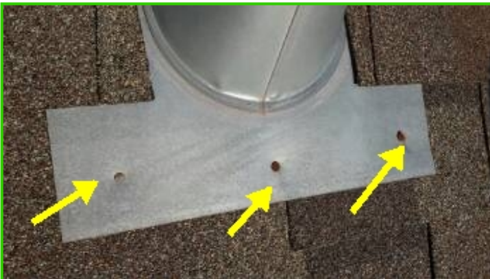
Seal with roof sealant. (NOT CAULKING)
