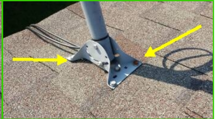
Seal with roof sealant. (NOT CAULKING)
