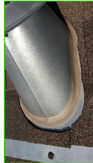
Sealant is in good shape.
