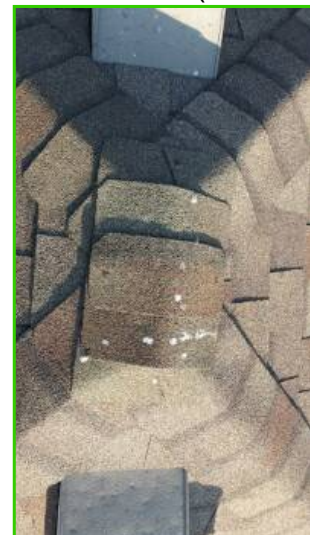
Seal nail heads at peak of roof.
