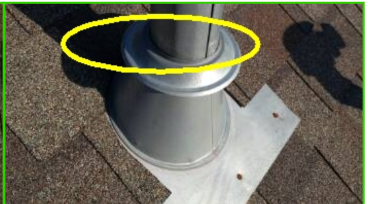
Seal with roof sealant. (NOT CAULKING)
