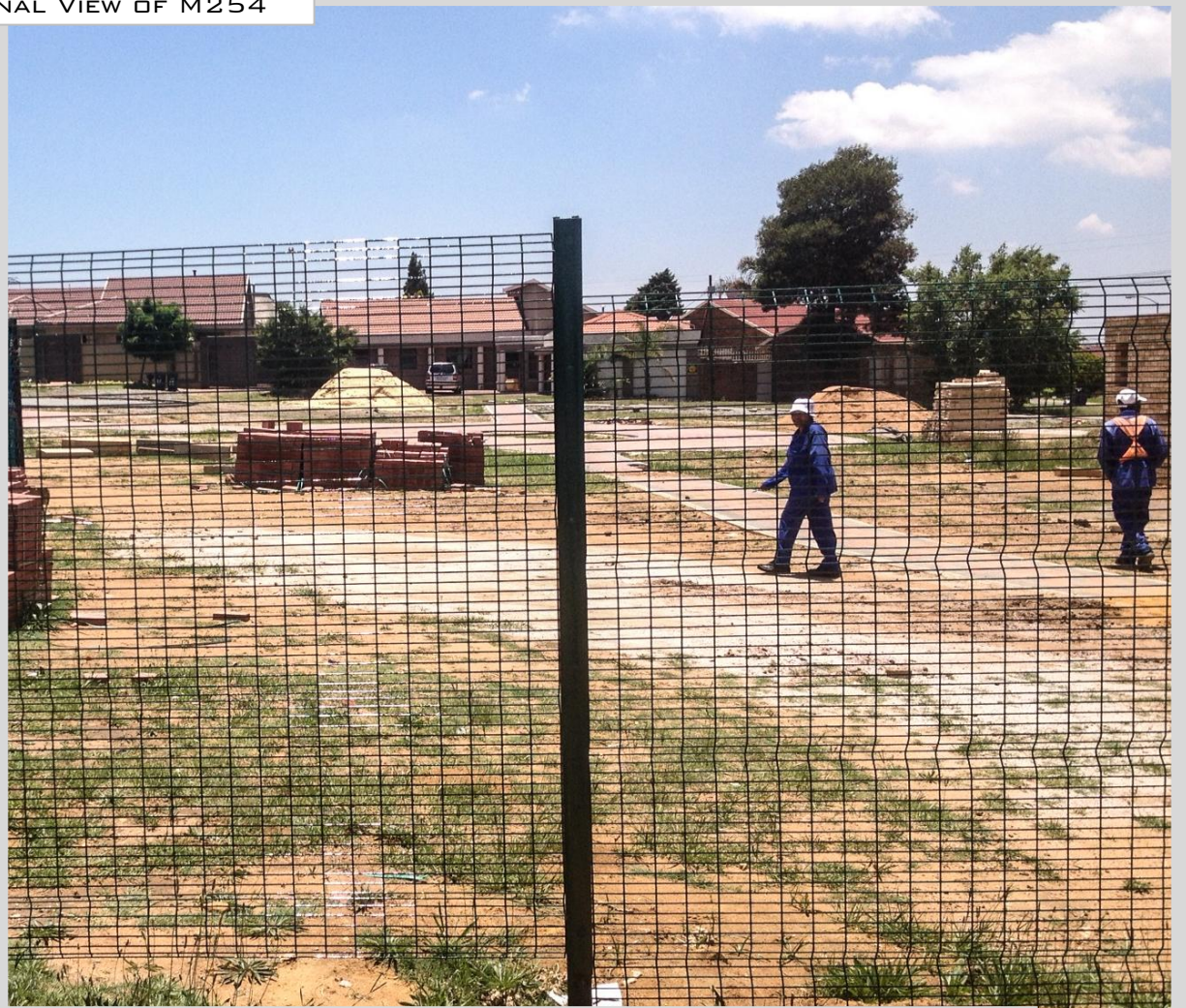
EXTERNAL VIEW OF M254
