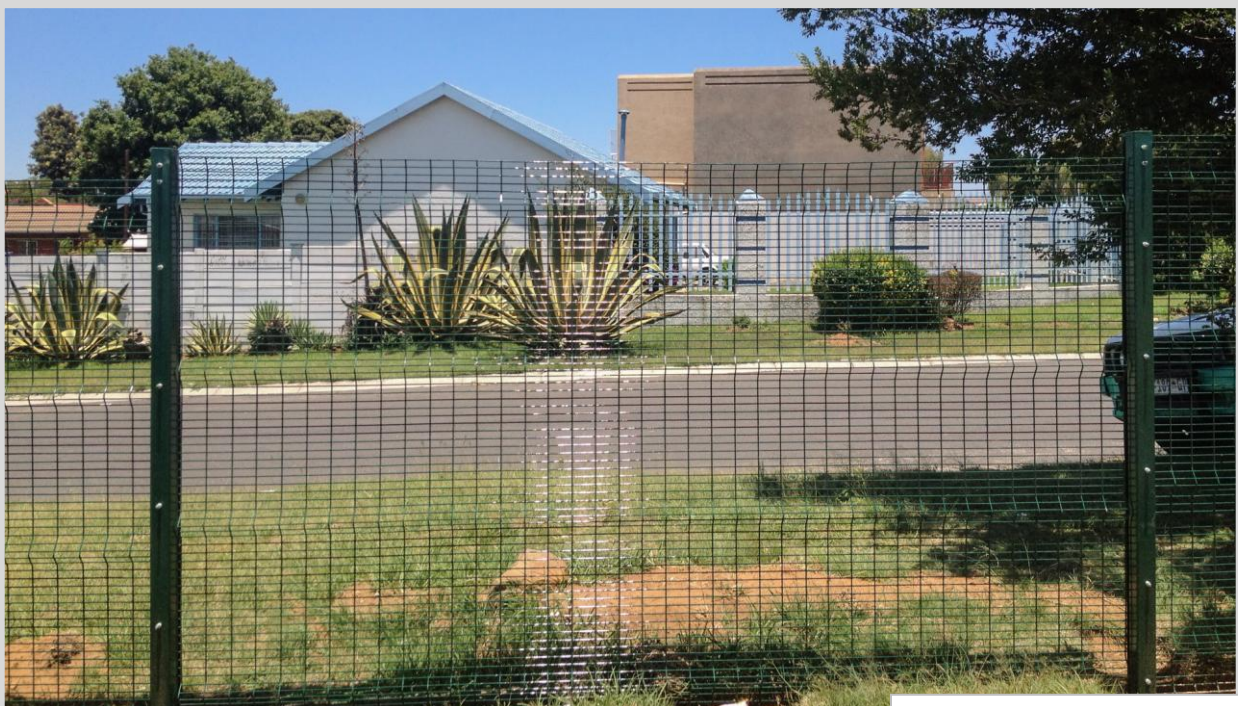
INTERNAL VIEW OF M254
