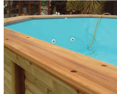
Once constructed, add in the liner and fill with water
