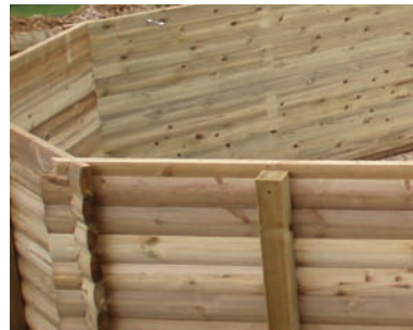
Build the wooden surround
