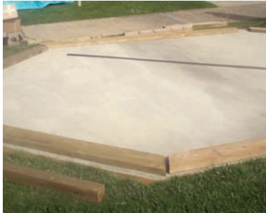
Concrete level base
