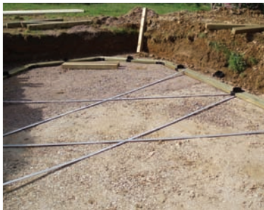
Dig the hole and prepare a flat base
