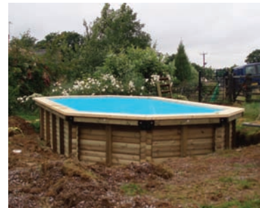
Once constructed, install the liner and landscape the garden
